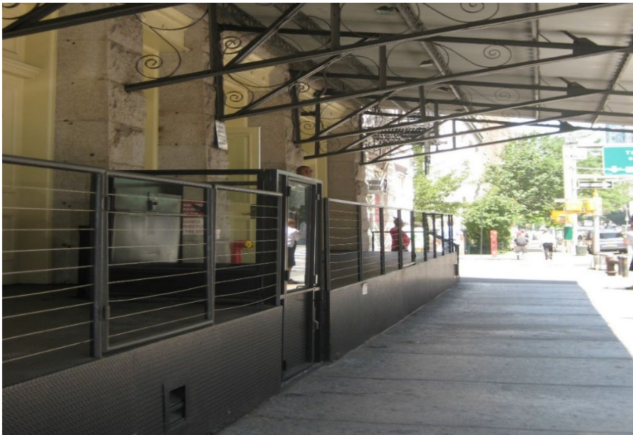
Figure 6. Platform lift with clear glass finished to match the adjacent building finishes
