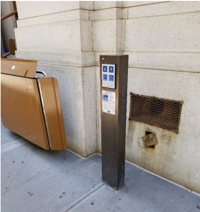
Figure 8. Actuator installed on a free-standing post.
