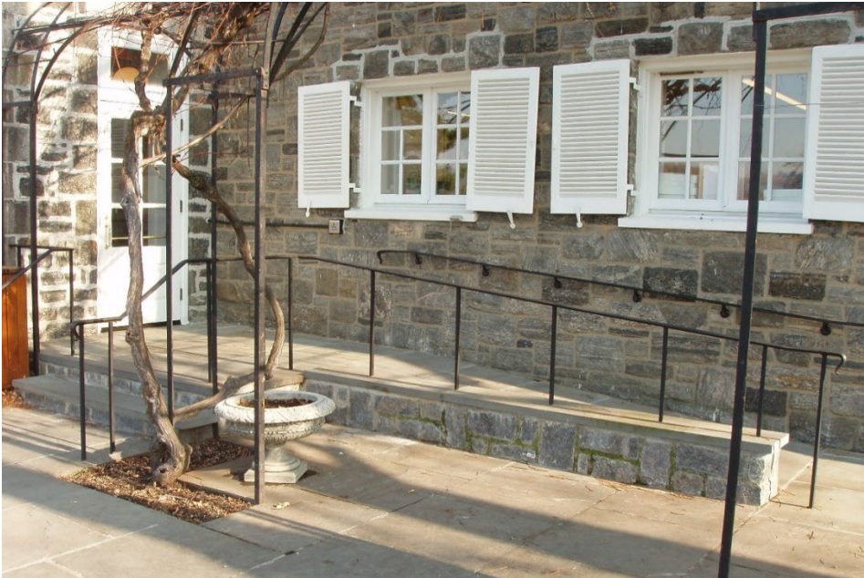
Figure 2. Ramp installed at a primary entrance with materials matching the historic building
