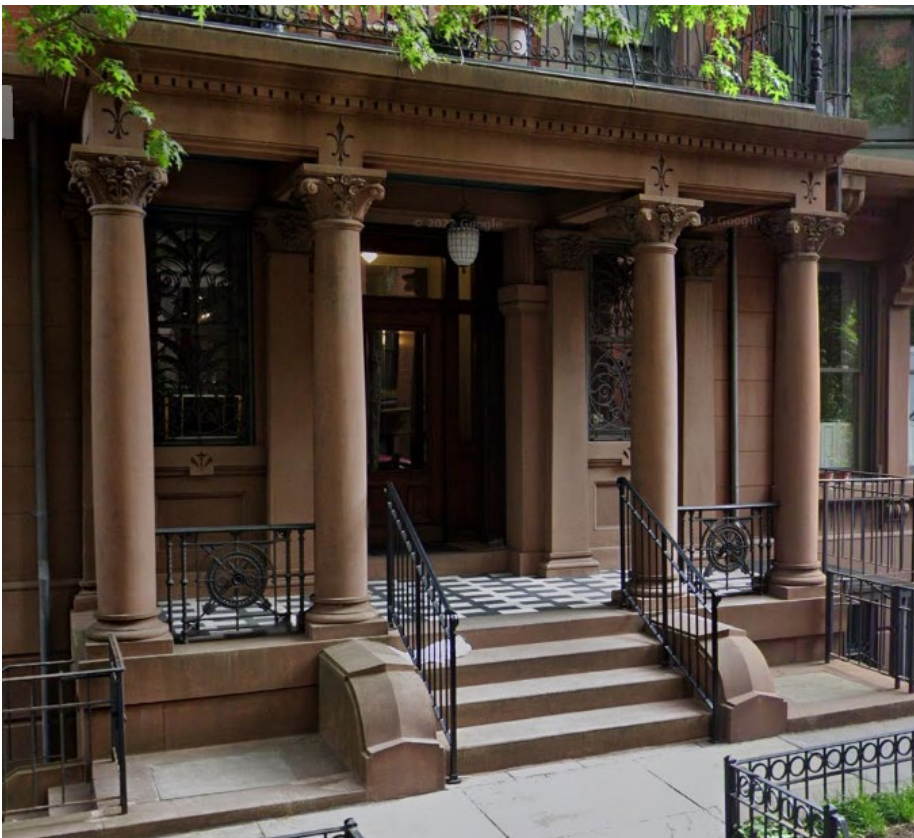
Figure 7. Before (top) and after (bottom) showing simply designed handrails installed at stair treads.
