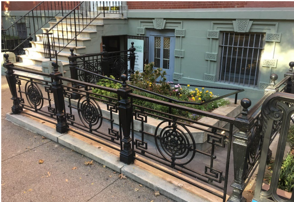
Figure 4. Ramp installed within an areaway
